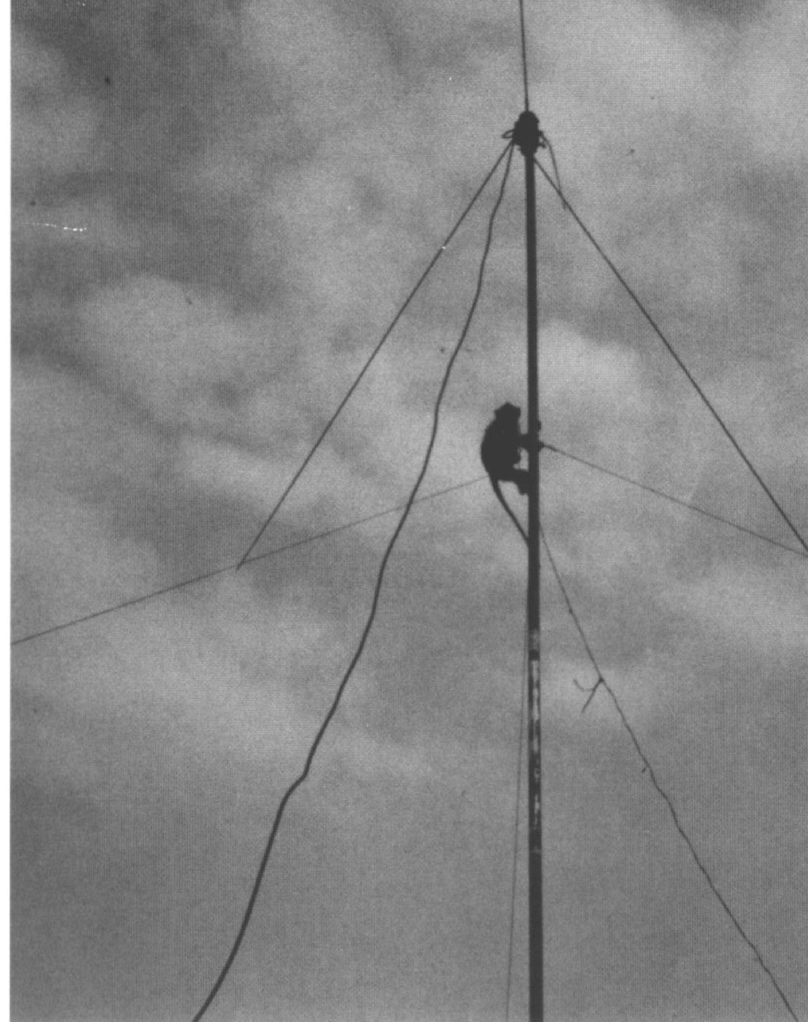
An unknown LRRP radio relay team member has climbed up the antenna mast to make last minute adjustments to Sgt Looney's equipment. The mast was held steady by two lines. The heavy line coming down was the transmission cable. (John Looney)
