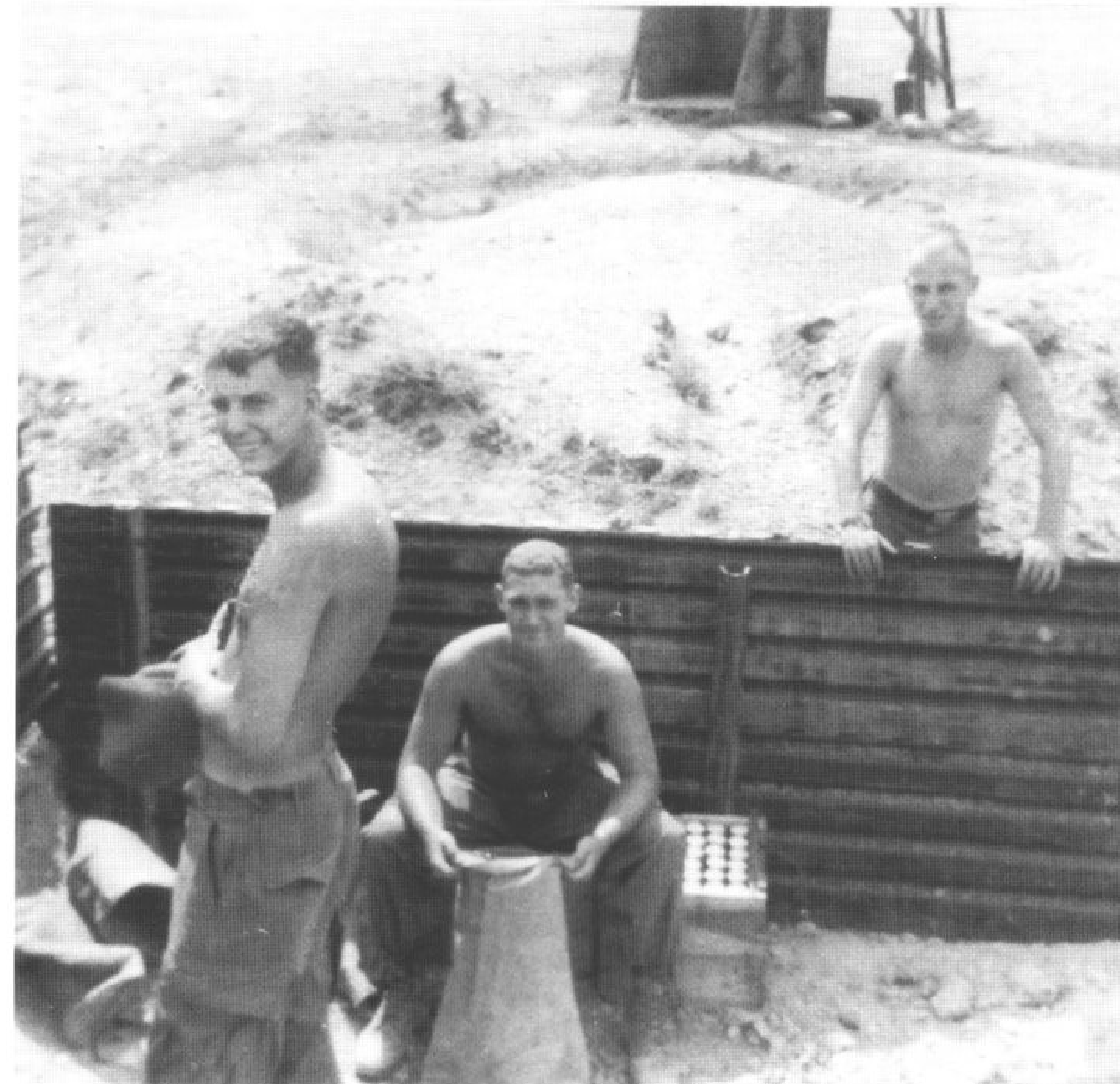
SSG Philip Byron , SP4 Evans, PFC Munoz building sand bag and sheet metal bunkers. The Army can always find constructive work for LRRPs between missions. Building bunkers and filling sandbags were the two most boring details we had; but when the B-40 rockets rained in we were very happy to have spent the time. Steel runway planking and sand bags were the building material of choice. (Author)
