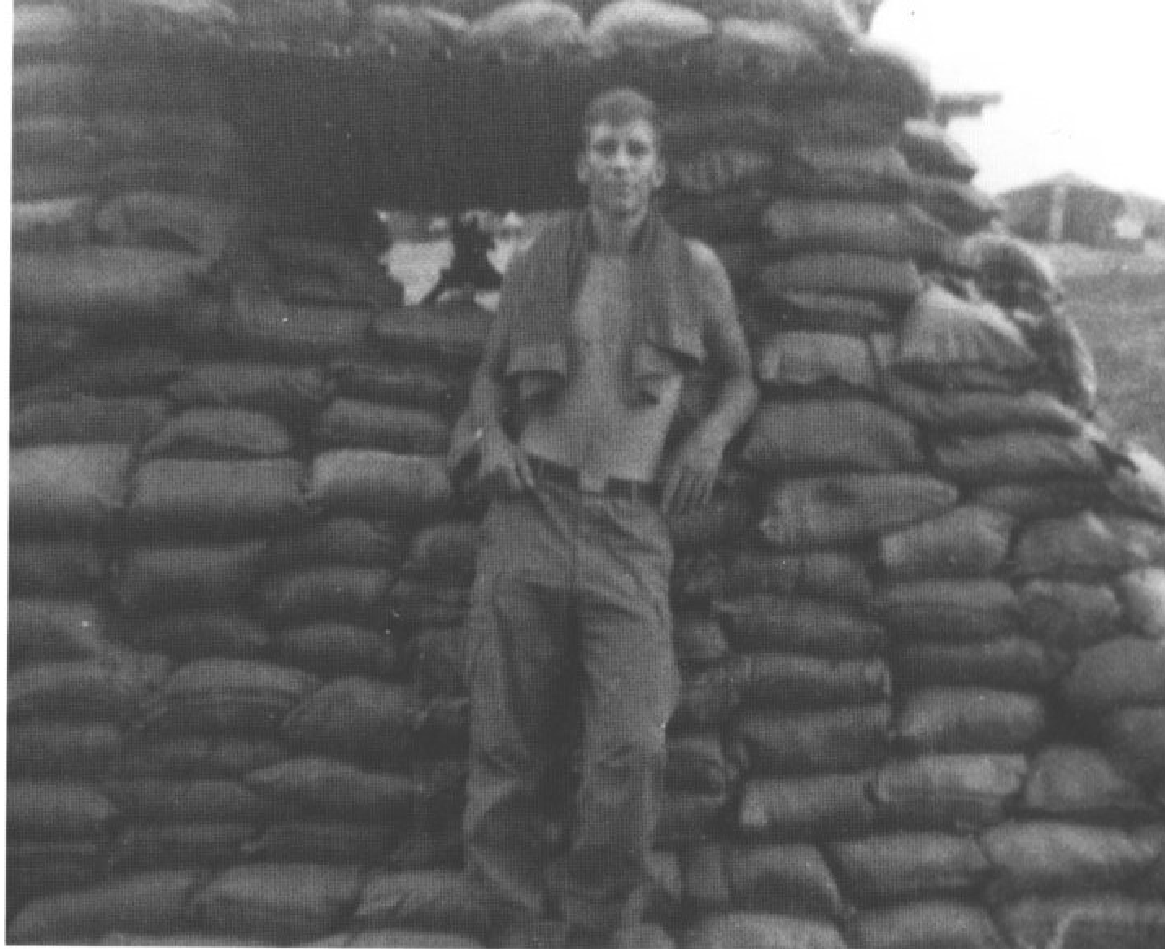
One of the machine gun bunkers we built in our sector of the base camp defensive perimeter. The opening in the center is the firing port for an 7.62MM M-60 machinegun. (Author)
