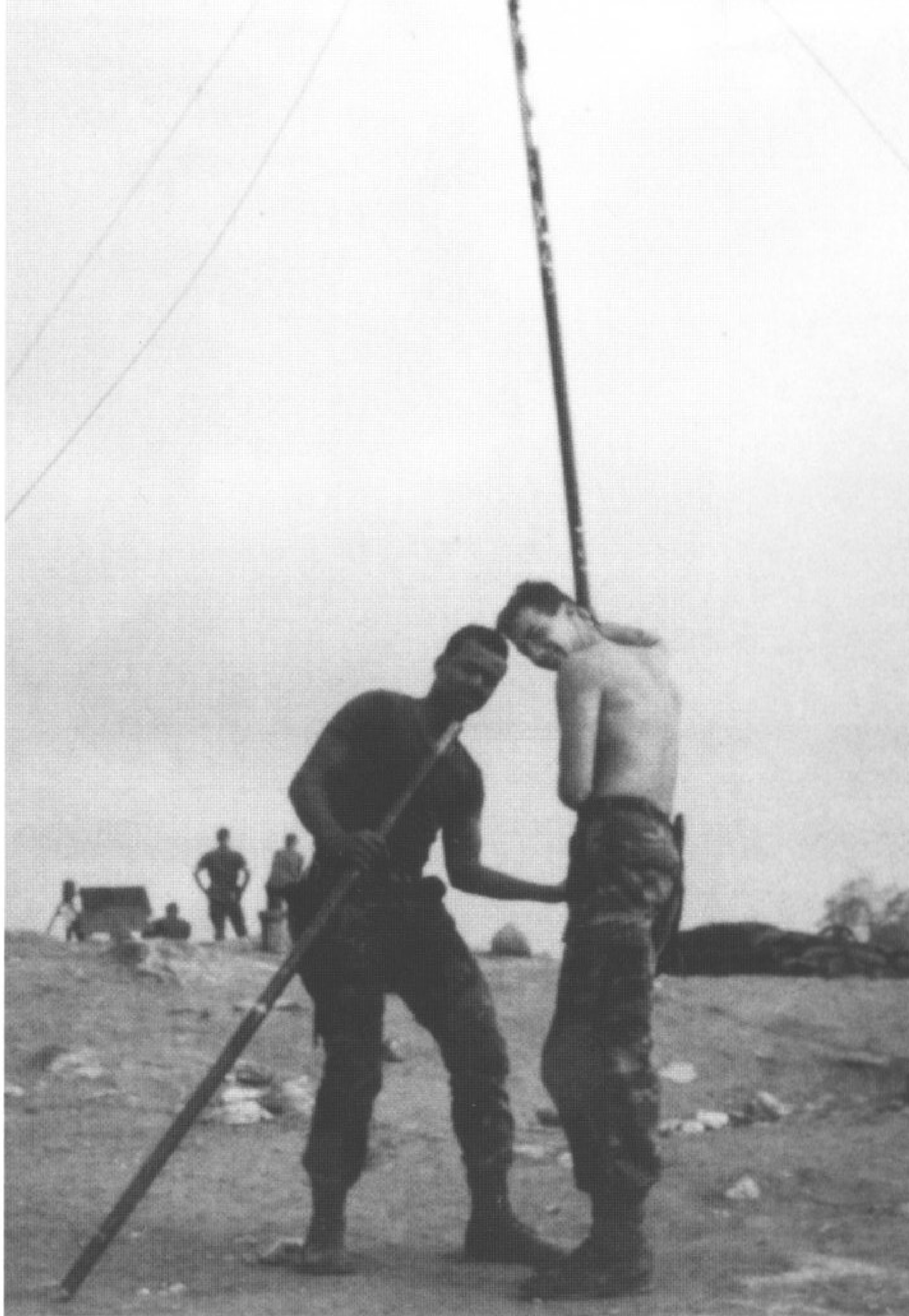
SGT John Looney and one of his team members putting up the AN-986A/6 antenna mast at a fire base before the patrols are inserted into the area of operations (AO). The radio relay would go out one day before a mission was started, to get set up and be ready to receive messages at the time of insertion. (John Looney)
