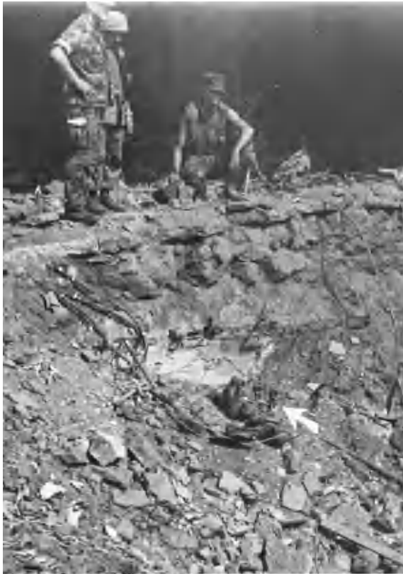
USMC Photo by SSgt Robert E. Kline A view of the crater made in the first floor of the BLT headquarters building by the explosion of the truck bomb which devastated the structure on 23 October 1983. The arrow points to a crankcase, all that remained of the truck after it was detonated.
